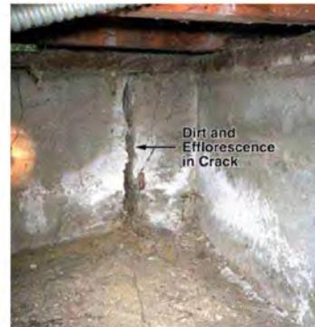
Dirt and efflorescence indicates age of foundation wall crack earthquake damage) [Exponent].
