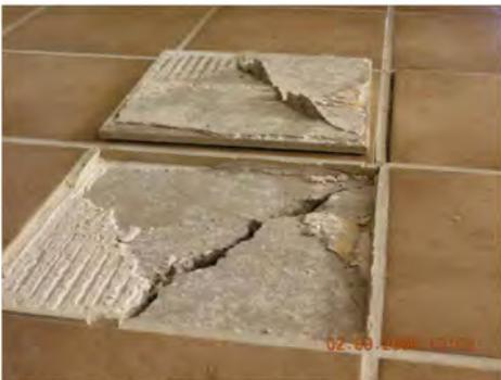
36. Setting mortar that had flowed into an existing slab crack that remained bonded to the backside of a ceramic tile when the tile was removed, a clear indication that the concrete slab was cracked when the tile was installed [Exponent]. <sup>35</sup>
